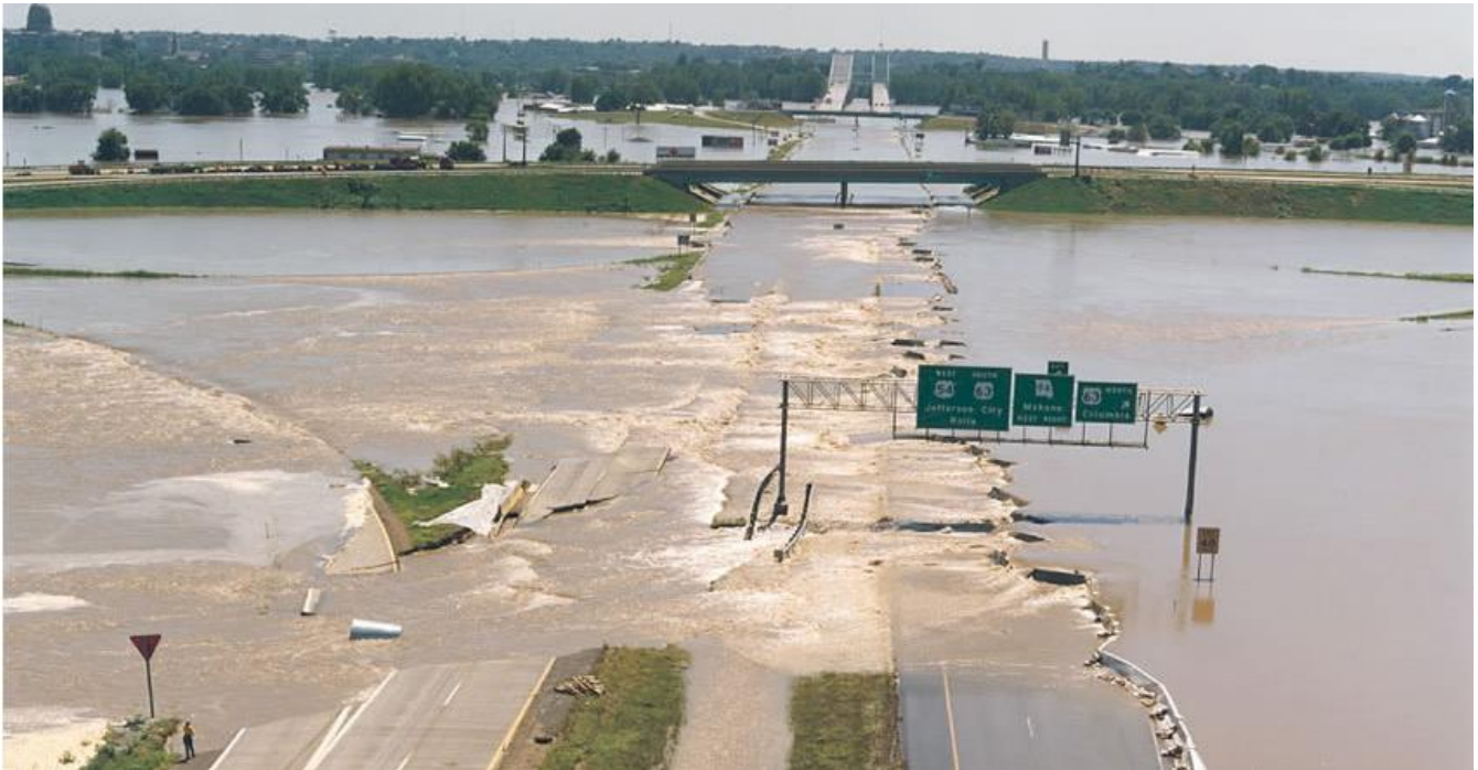
Figure 2. Photograph of Floodwaters During 1993 Midwest Flood (from Interagency Floodplain Management Review Committee, 1994)
